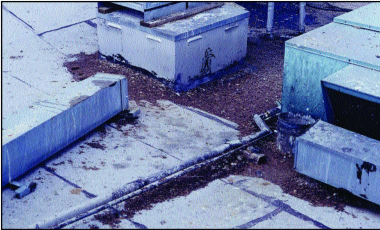
*Pigeon droppings, carcasses & nesting materials are heavy and can clog drains on roofs. This roof could collapse if water does not drain off properly and gathers. Droppings coming off the edge of these roofs and make a mess on the sidewalk below.*
