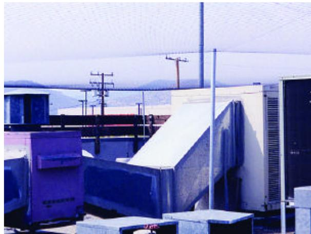
StealthNet protects HVAC equipment — StealthNet is an effective solution for Woodpecker problems
