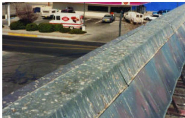
Roof and rain gutter damaged by bird droppings
